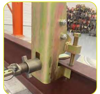
Stanchion installation complete
